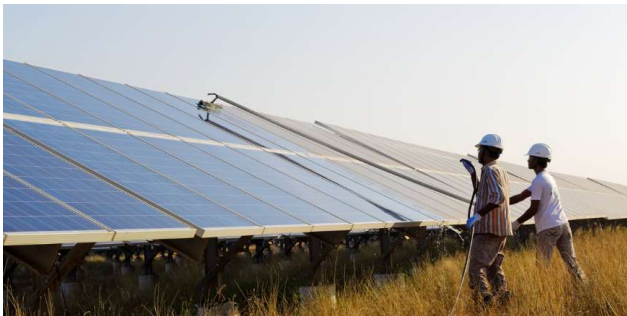
End-to-end project management
